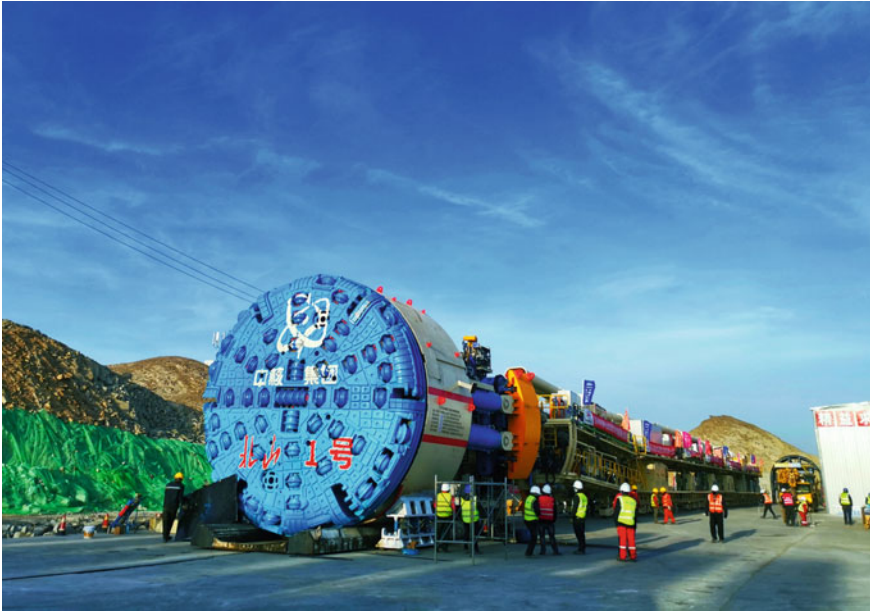
Fig. 2.13 The assembled TBM “Beishan No. 1” at Beishan URL
