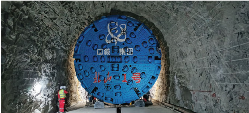
Fig. 2.14 The TBM “Beishan No. 1” in the ramp
