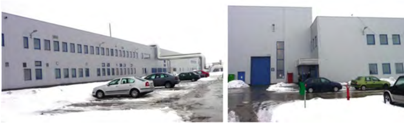
Fig. 4. Photos with case study building (difference in height between production unit and warehouse is visible in the right photo).
