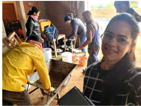
Fig. 8. Production of blocks using Ulva at a local company ‘SOIB’.
