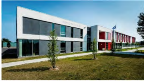
Fig. 1. Studied school building, Horizon-du-Lac (near Montreal, Canada) [16].
