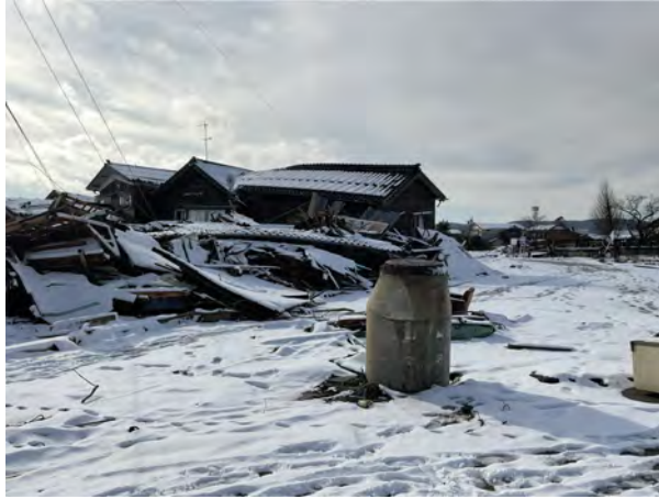
Fig. 4. Collapse of classical wooden Japanese houses due to ground motion, tsunami and/or liquefaction caused by the 2024 Noto-Hanto earthquake. Note that the picture was taken by the second author.
