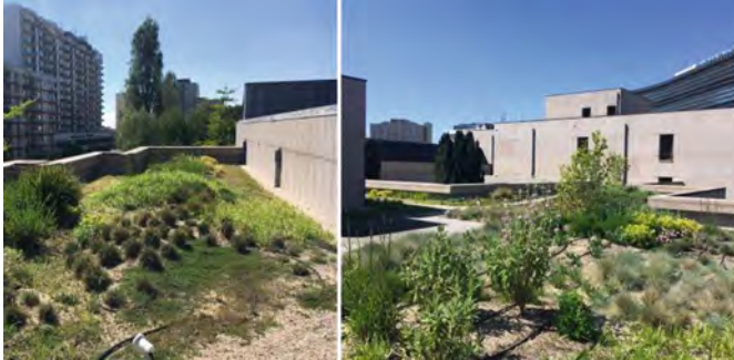
Fig. 3. Semi-intensive green roof implemented at Fórum da Maia, Maia, Portugal.
