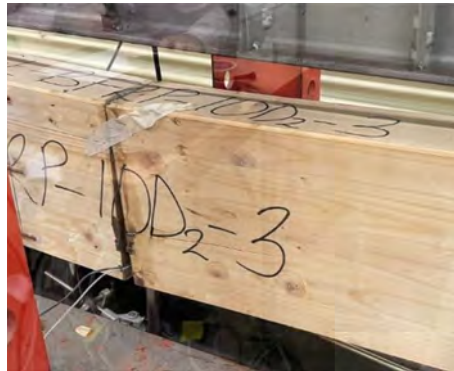
(b) 10 – D2 – 3: Debonding at the interface; pull-out of bars at tension zone; splitting at the soffit of the beam; splitting of timber at compression zone
