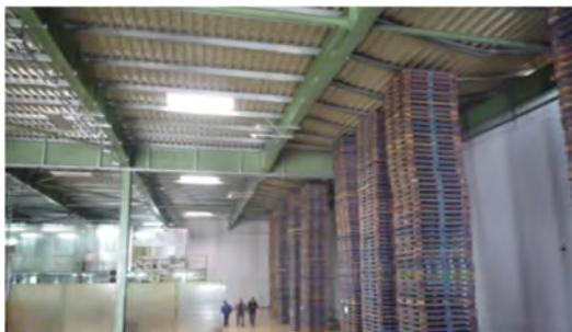
Fig. 7. Sandwich panels and purlins propped by wooden pallets.
