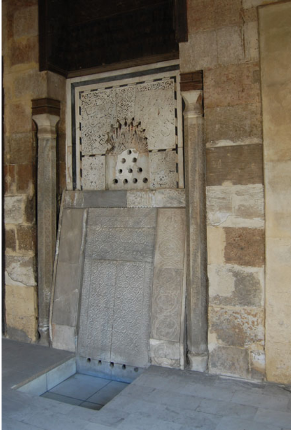
Fig. 3 Sabīl of Sultan Qāyṭbāy (interior). The finely carved marble slab (Ar: sālsabīl or shādhirwān ) where water was poured to be cleansed and cooled down before being offered to passers-by (Angela Isoldi)
