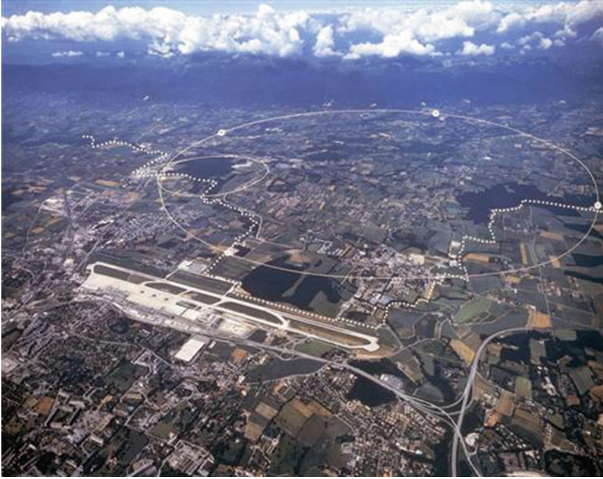
Fig. 10.3 An aerial view of CERN and its surroundings, showing the position of the LEP ring. The runway of Geneva airport gives an idea of the scale (©CERN, All rights reserved).
