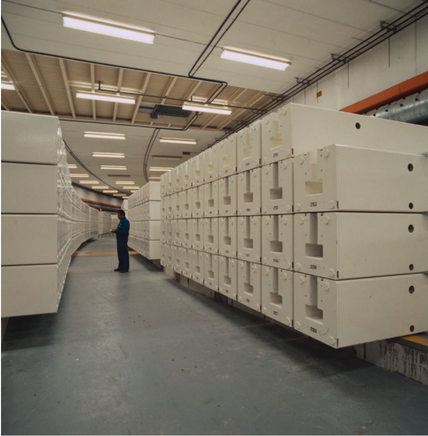
Fig. 10.4 LEP's innovative so-called concrete magnets stored in the ISR tunnel awaiting installation. This was the first time the Laboratory had gone into mass production at this scale (©CERN, All rights reserved).
