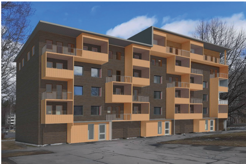
Figure 3. Representative image of wooden facade renovation.
