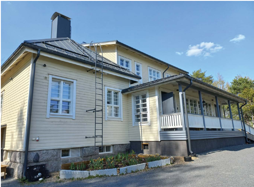
Figure 5.12 Pöllölä building after renovation work completion (authors' own)
