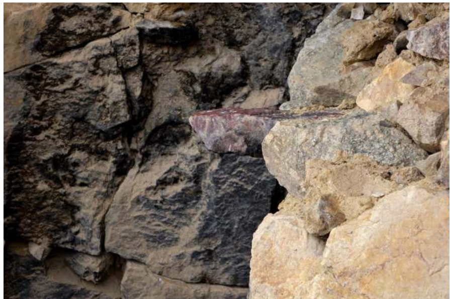
Figure 65. One of the in situ corbels belonging to a building in the upper tier. This is a tell-tale sign that the structure and others in the upper residential complex possessed an all-stone roof raised in the archaic manner.
