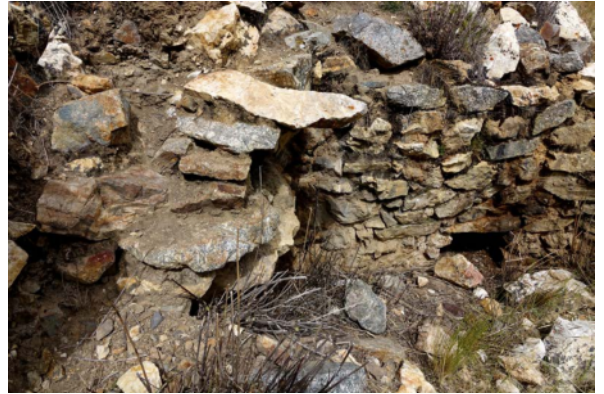
Figure 68. East room of the middle tier. Corbels protruding from the rear wall and a niche at ground level are visible in the photograph.
