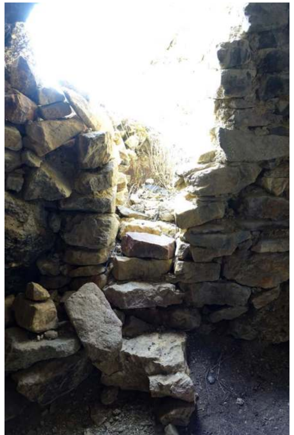
Figure 49. The entrance and façade of cave 2 as seen from the interior.
