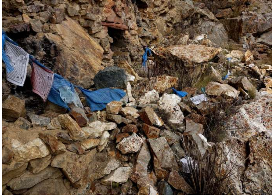
Figure 64. Highly degraded ruins of rooms belonging to the upper tier of the upper residential complex. Note the entranceway to cave 4 above the ruins.
