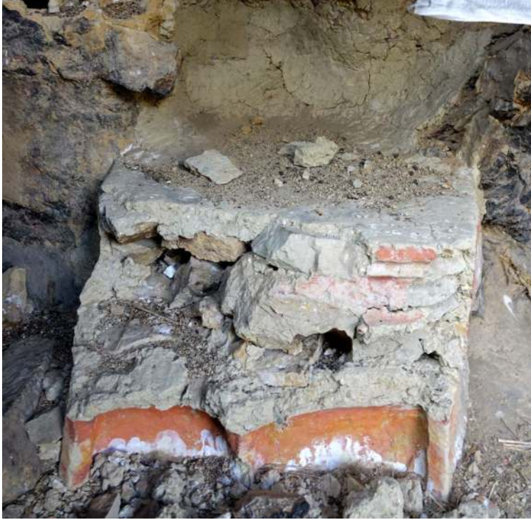
Figure 59. The masonry and adobe platform, with traces of orange (ochre) and white pigments on the exterior faces, which was built into cave 3 at Mgon bdag.
