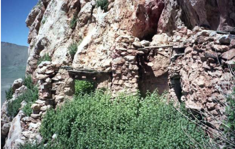
Figure 111. One of the cliff shelters in Rdzong dkar po. This multi-roomed structure was split between two levels. Note the stone lintels and corbelling.
