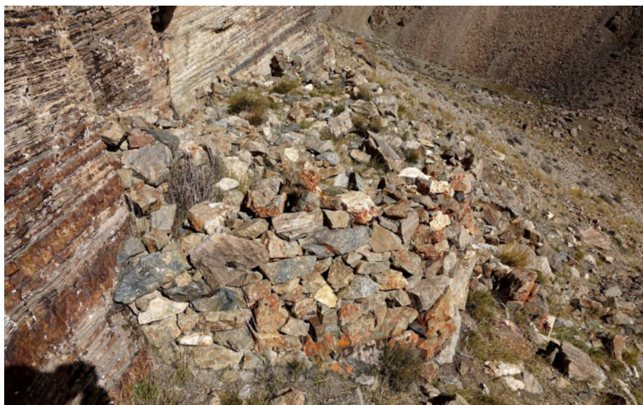
Figure 81. Wall footings and a revetment at the foot of the grey outcrop residential complex.
