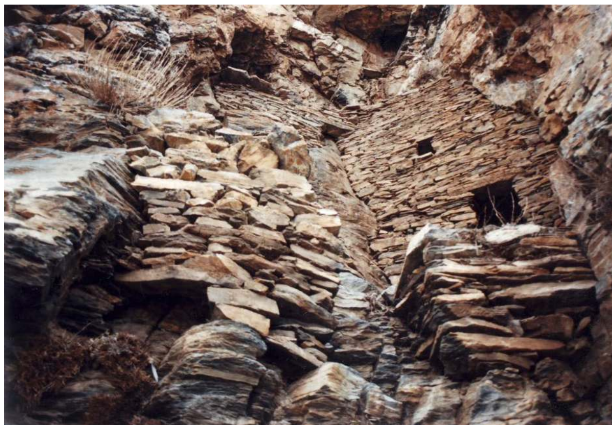
Figure 123. The three-storey masonry façade of a cliff shelter at Rdzong pi phi (S43). The upper portion of the façade encloses the cave that harbours most of the rock art at the site. The entrance to the cave is visible on the right side of photograph.
