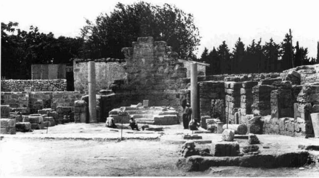
Illus. 87. Cyrene: East Church, west apse and part of nave.
