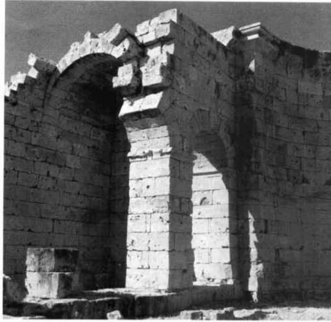
Illus. 137. Ptolemais: West Church, barrel vault of north arcade, with transverse rib.
