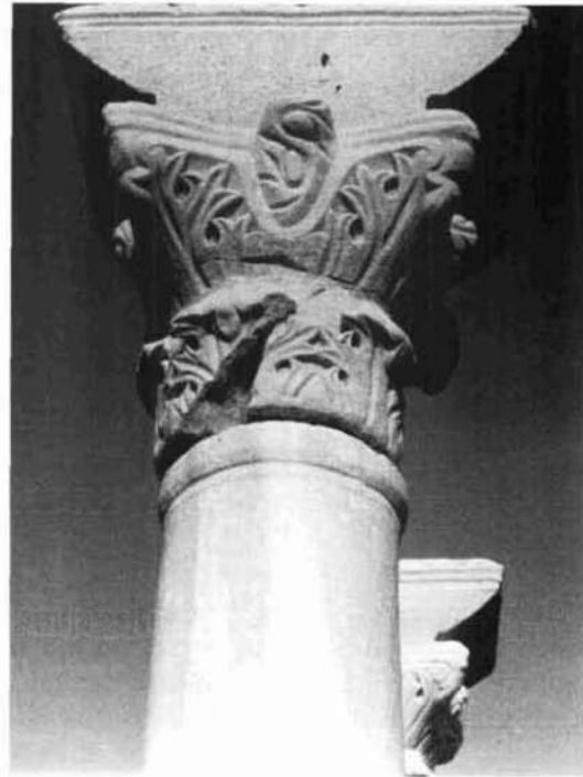
Illus. 188. El Atrun: West Church, marble column with capital and impost block from the nave colonnade.
