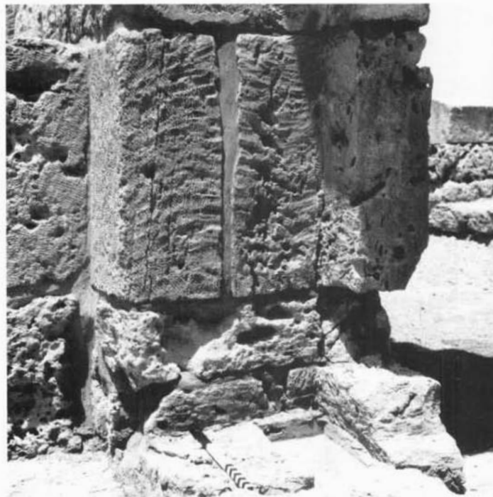
Illus. 64. Apollonia/Sozusa: 'Palace' Chapel, main entry from peristyle court
