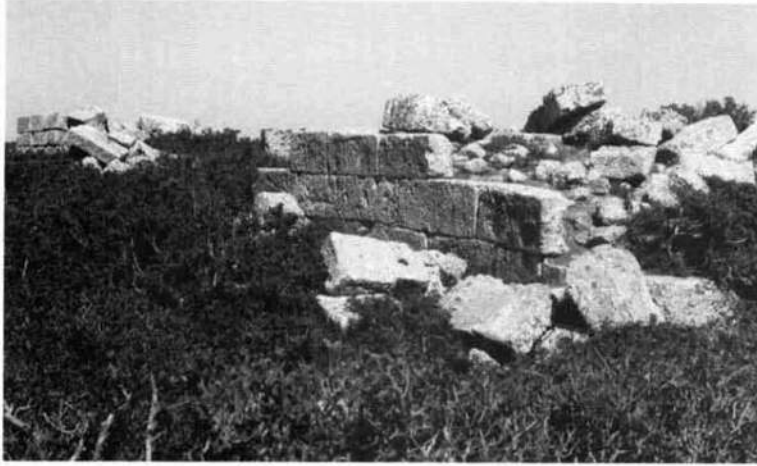
Illus. 313. Umm Heneia el Garbia: the church, outer face of perimeter wall.
