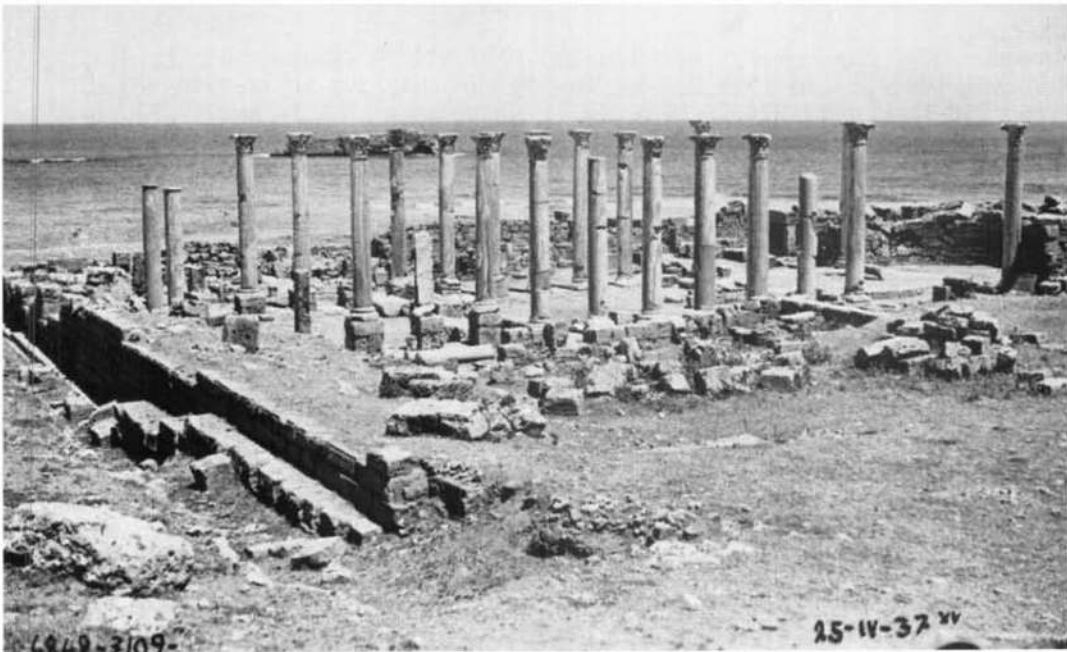
Illus. 5. Apollonia/Sozusa: East Church, seen from the south-west after reconstruction.
