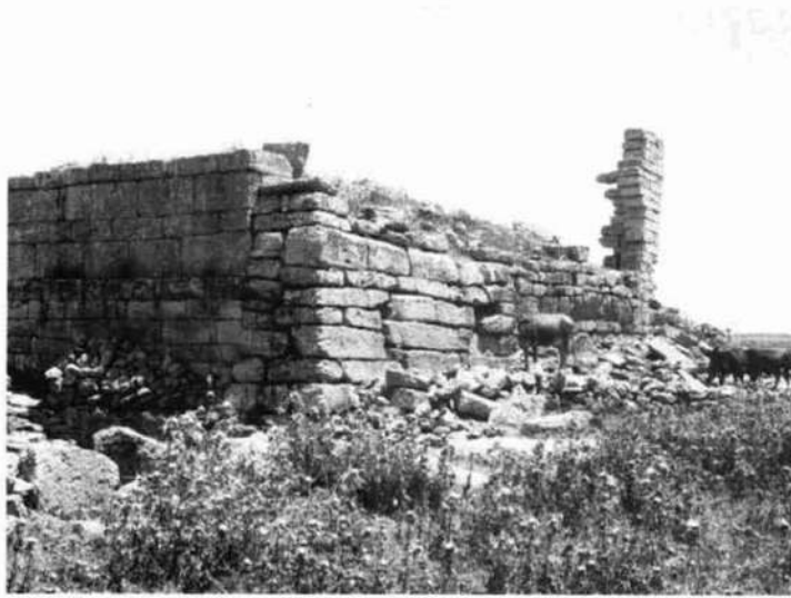
Illus. 260. Mtaugat: the church, revetment along west wall.
