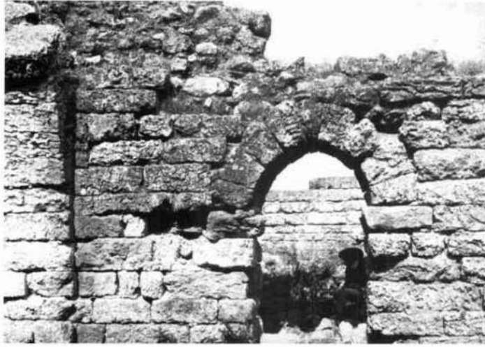
Illus. 321. Zawiet el Argub: building of controversial purpose, door from 'chancel' into Room NE1.
