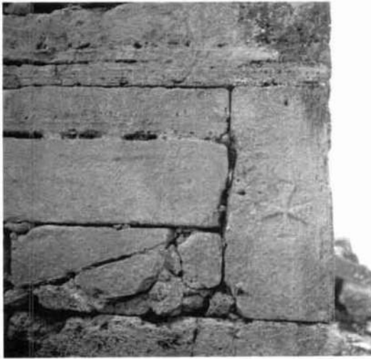
Illus. 232. Gasr Silu: gasr, cross on the north-west corner stone.
