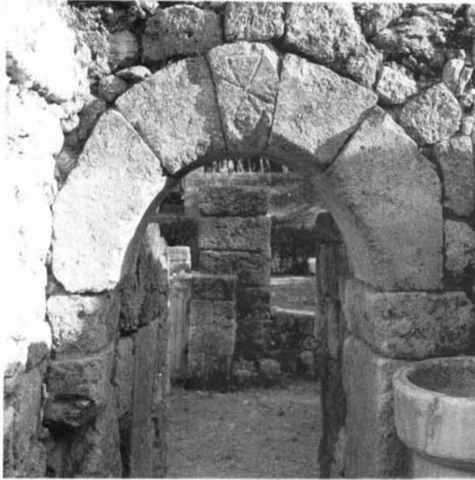
Illus. 100. Cyrene: East Church, archway into the north aisle.
