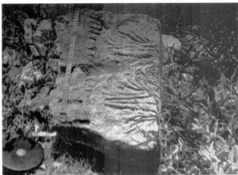
Illus. 332. Gasr Asceisc: pilaster capital fallen from fortified Christian building.
