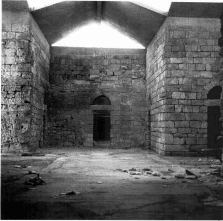
Illus. 216. Gasr el Lebia: West Church, west doorway.
