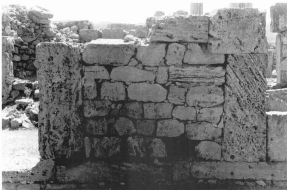
Illus. 10. Apollonia/Sozusa: East Church, orthostats used in faced-rubble construction.
