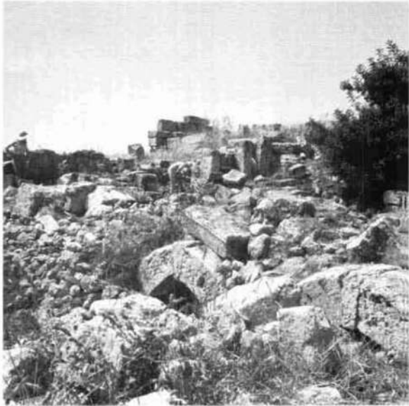
Illus. 249. Messa: the church, north nave arcade.
