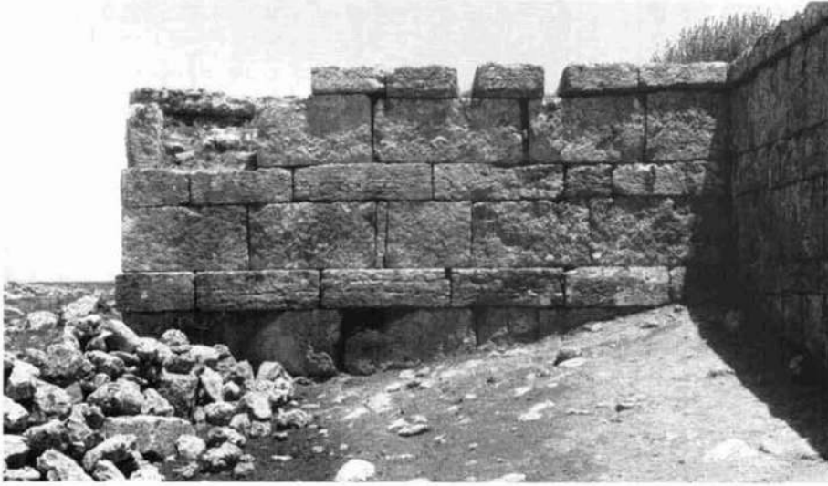
Illus. 262. Mtaugat: the church, masonry of projecting north-east wing.
