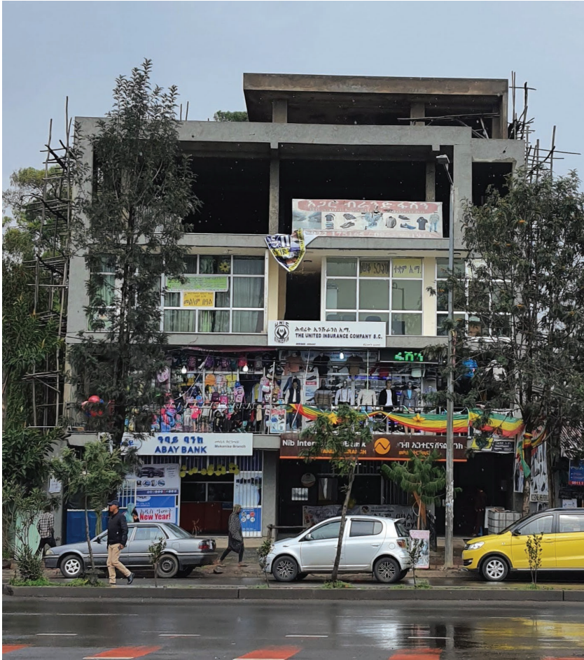
Figure 3.3 Iddir-owned mixed-use building with upper floors incrementally constructed so that one or two floors can be used for income generation ( photos by the author ).
