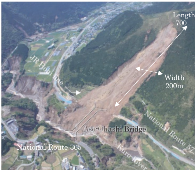
Fig. 23 A slope failure induced by the mainshock near the Aso-Ohashi Bridge (Modified from the Kyushu Regional Development Bureau, MLIT 2021) (Fig. 10 in Higaki et al. 2023)
