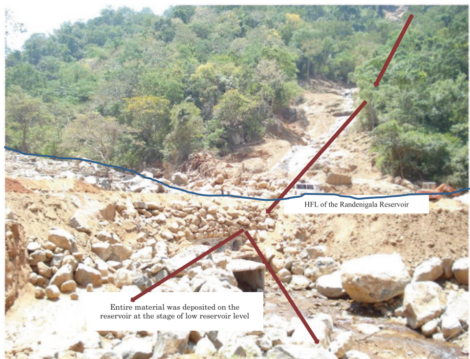
Fig. 2 Roakslide was initiated from the upper mountain region of the reserved forest towards the reservoir second largest reservoir of the Randenigala Hydroelectric Power Project (Photo by Gunathilake, A.A.J.K.)
