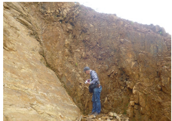
Fig. 6 Failure along major rock-slope joint plane (Photo by Dias, A.A.V., July 2017)
