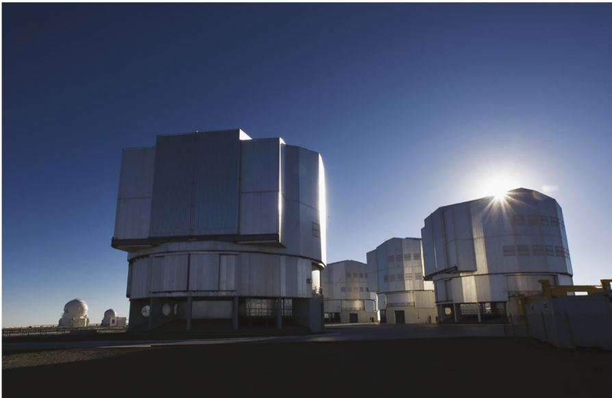
Figure 8.2b The Very Large Telescope on Cerro Paranal in Chile, consisting of four 8.2m aperture telescopes
