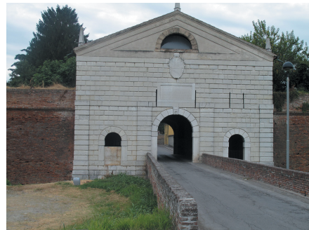
Figure 4: A Renaissance-style 'imperial' porta served as the principal access point to the 'ideal city' of Sabbioneta (near Mantova in Italy) built by Vespasiano Gonzaga Colonna in the late sixteenth century. In the central axis of the gate, the duke's arms appear in the medallion above a dedication to his overlord, Emperor Rudolph II, on the rectangular panel. Picture Allain Rouiller 2010, released under a CC-2.0 license.
