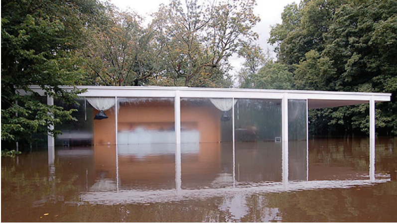
FIGURE 2.2 The Farnsworth House flooded by the nearby river
