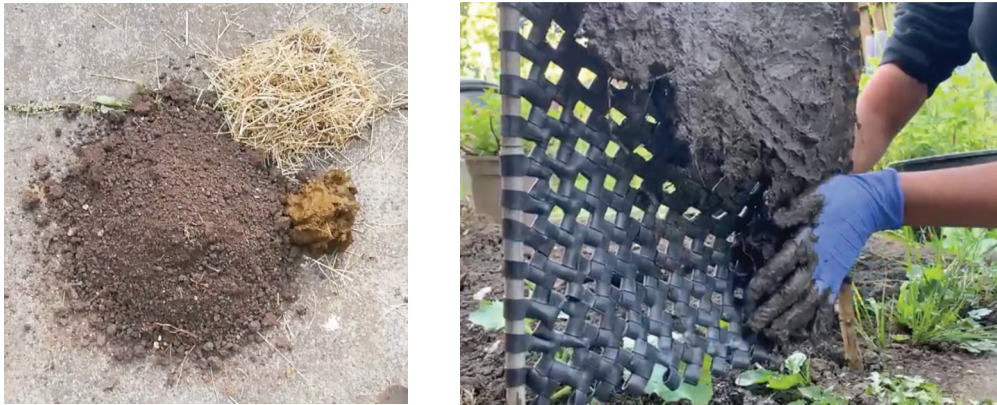
FIGURE 8.5 Traditional loam mixture: soil with straw and dung | application
