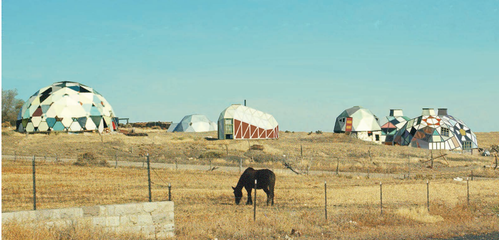
FIGURE 6.8 The inherently highly ideological re-use language of the DIY geodesic domes fabricated from materials such as salvaged car bonnets at Drop City (1965–1973).
