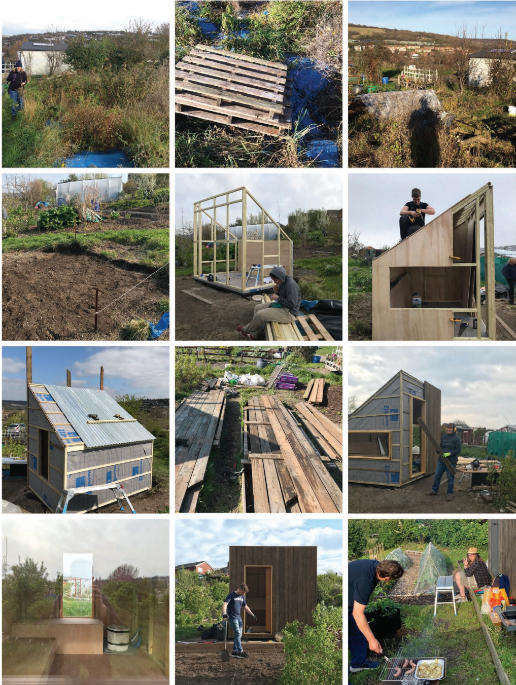
FIGURE 0.5 The shed build process (2018–19)
