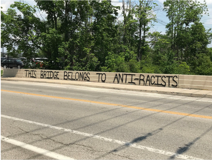
Figure 9.1 The eastern-facing wall of ‘Graffiti Bridge’. © Fernando Orejuela.
