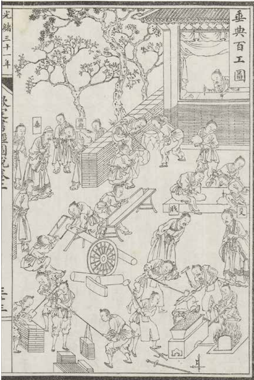
Figure 2. Workers of various trades: sawyers, bricklayers, blacksmiths, and long-gowned official supervisors. Chui dian baigong tu 垂典百工圖 [Illustrations for handing down the methods of the hundred trades]. In Sun Jia'nai 孫家鼐, Li Xisheng 李希聖, Zhan Xiulin 詹秀林 and Zhan Bukui 詹步魁, Qinding Shujing tushuo 欽定書經圖說 [Imperially endorsed illustrations and explanations of the Book of Documents ] (Beijing 北京: [Neifu 內府], 1905) 2/33a. Reproduced with permission of Staatsbibliothek zu Berlin – Preußischer Kulturbesitz, Germany.
