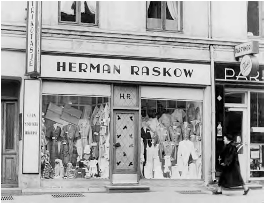
FIGURE 1.7 The knitwear and hosiery shop Herman Raskow at Hegdehaugsveien 26, Oslo.
