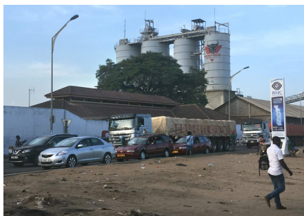
USINE HEIDELBERG CIMTOGO, LOMÉ, TOGO, 2018 [© ACML].
