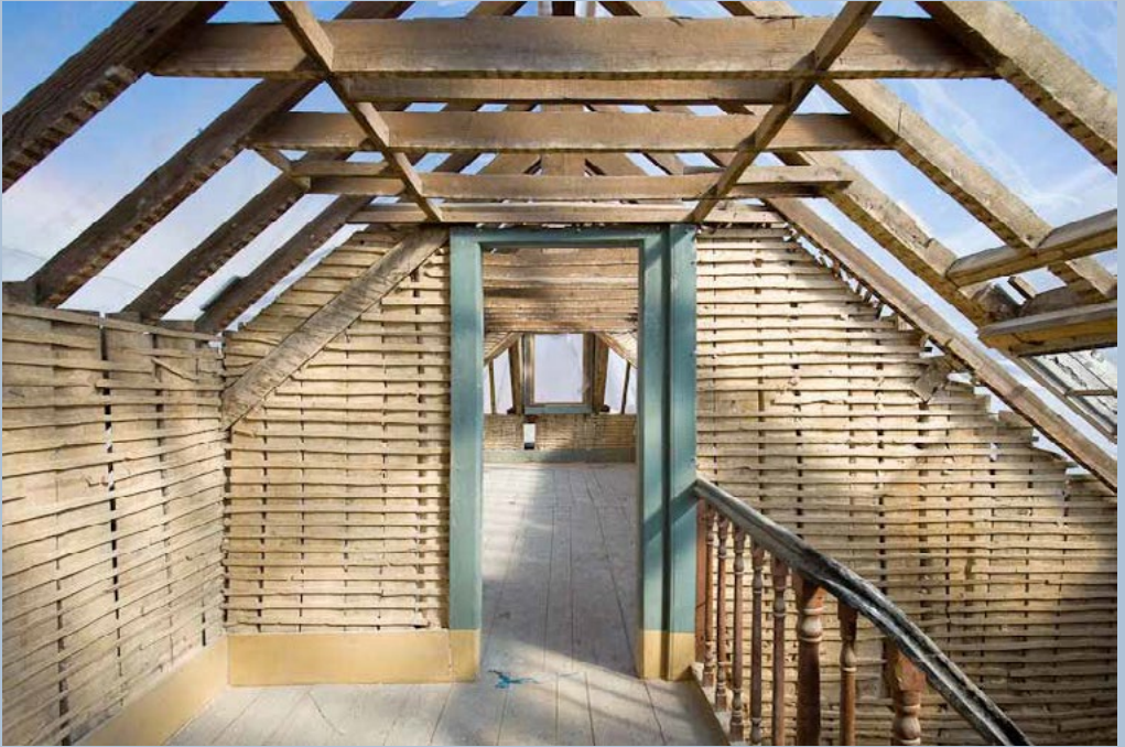
Top floor during renovation work
