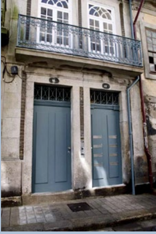
Street façade (photo | Pedro Camelo)
