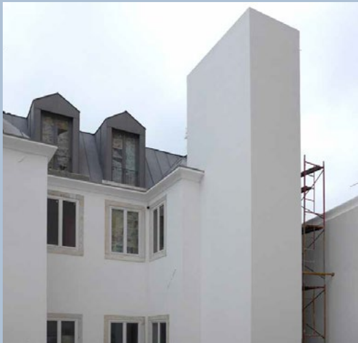
Courtyard façade and lift (photo | Catarina Wall Gago)
