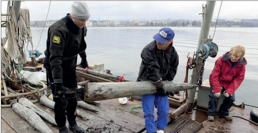
Fig. 3.3 Extraction of piles from the site of Plonjon (Image: Olivier Zimmermann).
