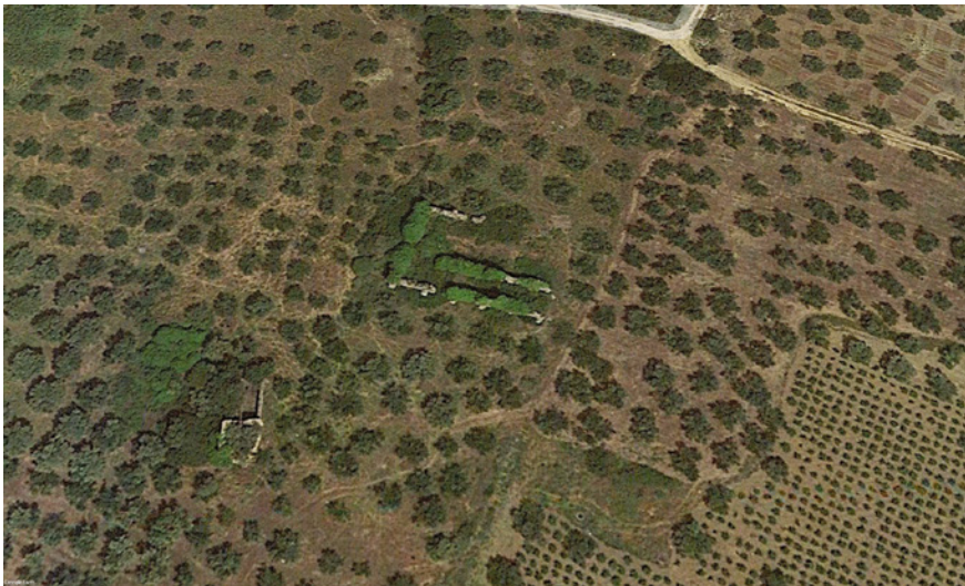
FIGURE 51 The building of Agioleos in its present state
