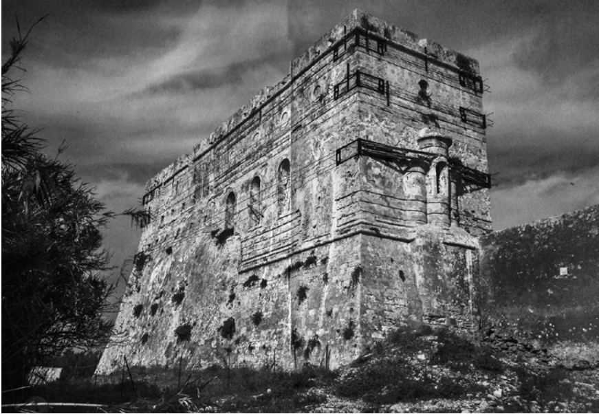
FIGURE 44 The east side of the tower and the apses of the katholikon of the monastery of Strophades
