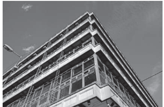
The FADU building follows the paradigm of the modernist movement. The design of the campus as a whole was entrusted to the architects Caminos, Catalano, Sacriste, and Picarel. This rectilinear building with its almost unbroken symmetry fits within the most orthodox streams of the modern movement. Repetitive lines of reinforced concrete and cantilevers form the exterior. They are separated by rows of rectangular glass windows framed with thin steel, creating a rigorous structure. The whole construction celebrates glass and concrete and lacks any ornamentation or color. Photo: Maya Ober.
