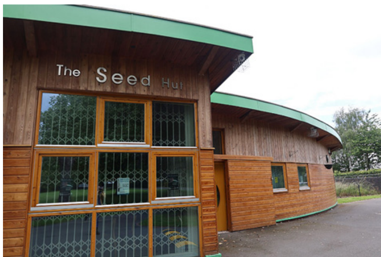
Figure 4.4 The Seed Hut was built as part of One Palfrey Big Local. It comprises rooms for activities, the project co-ordinator's office, a kitchen and toilets, 2021
