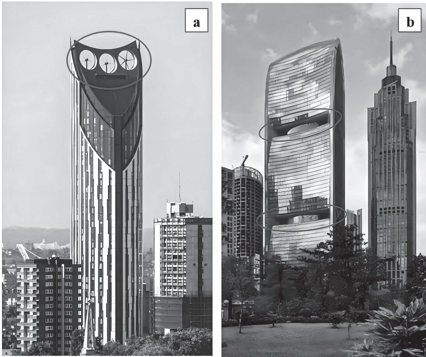
FIGURE 8.13 Wind turbines in buildings. (a) Strata Tower, 16 London. (b) Pearl River Tower, 17 China.
