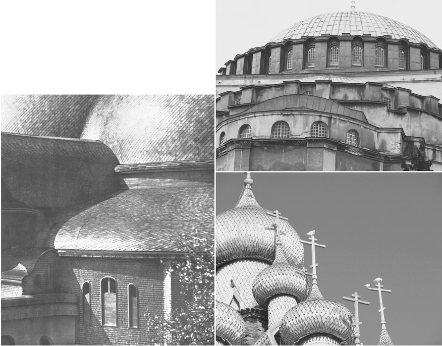
Figure 5: Norway slate of the First Goetheanum (Fig. 5a), domes of Hagia Sophia (Fig. 5b), and the Church of the Transfiguration of the Savior in Kizhi, 1714, layered with wooden shingles (Fig. 5c). Image Credit (5a): The Goetheanum Archive, Dornach, Switzerland, courtesy with support by Marianne Schubert, 1992; (5b): NGM, June 27, 2022, open access, photo: James L. Stanfield, clipped; (5c): Anna Sokolina personal archive.
