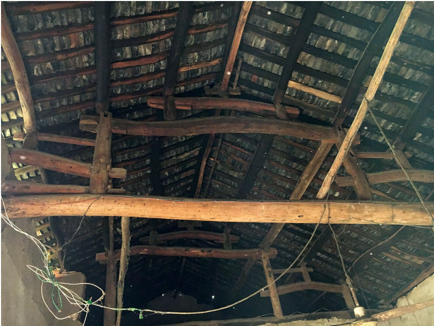
Plate 1.2 Two dragon-gate roof frames
