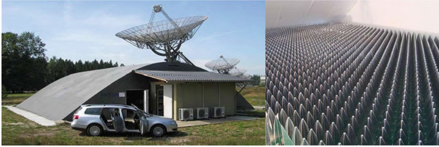
Fig. 6.30 Left: The EMBRACE station under a large, curved radome. Right: Inside the radome. Shown are the aluminium Vivaldi radiators in a dual polarisation configuration of about a quarter of the array. Credit: ASTRON
