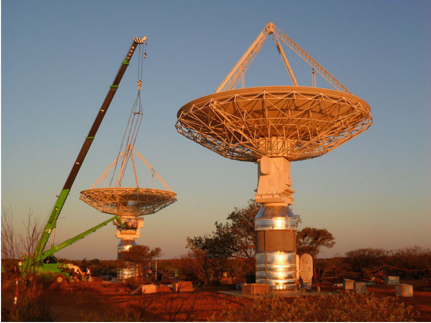
Fig. 6.10 The ASKAP antennas under construction. The third axis of rotation is located just under the reflector. Credit: CSIRO Radio Astronomy Image Archive CRAIA-SKA011
