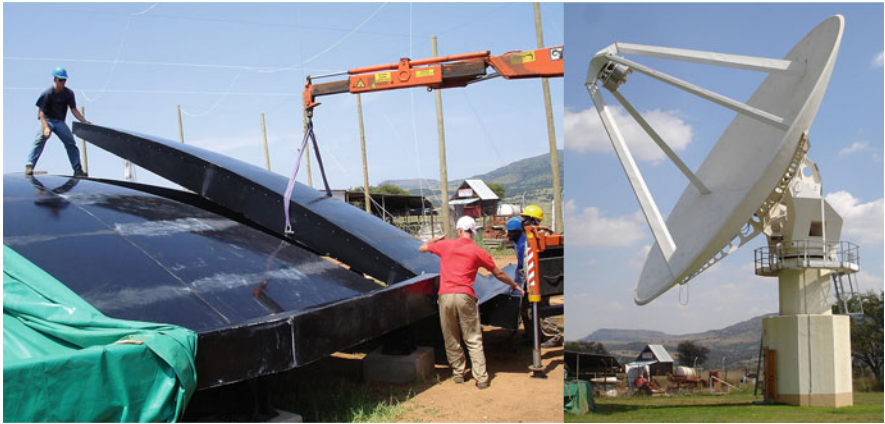
Fig. 6.12 Left: The XDM telescope mould under construction at Hartebeesthoek Radio Astronomy Observatory in South Africa in 2007. Right: The XDM with all subsystems installed, integrated and tested in 2009. Credit: South African Radio Astronomy Observatory (SARAO)
