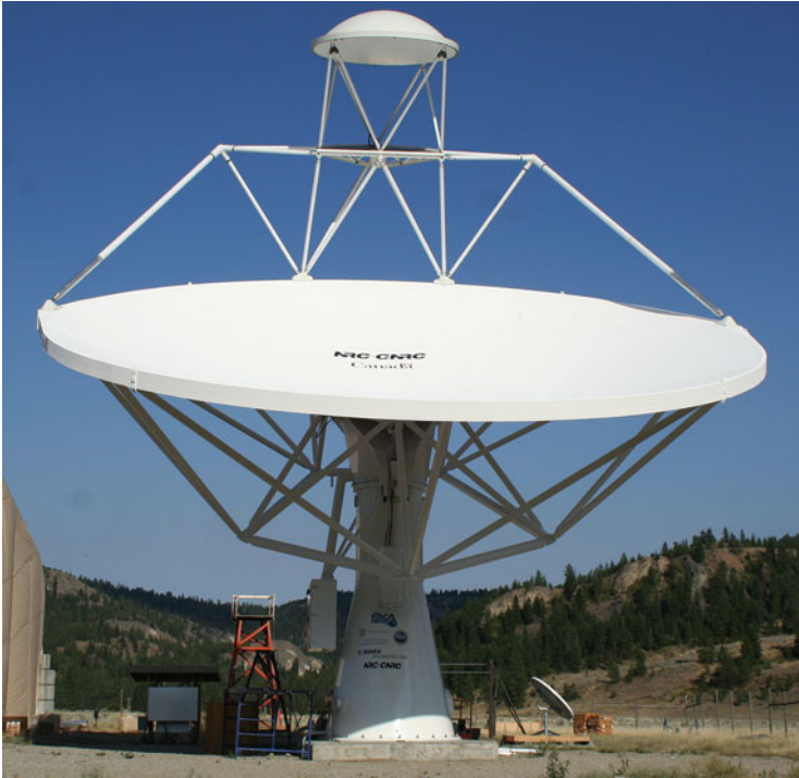
Fig. 6.18 The DVA-1 dish, after repairs and shortly after the sub-reflector was mounted. Credit: The National Research Council of Canada
