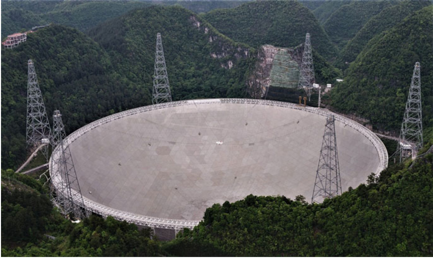
Fig. 3.8 The 500 m diameter FAST dish in Guizhou Province in China. It is an active-surface spherical dish with collecting area of 196,000 m 2 located in a karst depression, and operates at frequencies from 70 MHz to 3 GHz (with plans to upgrade to 8 GHz in the future) (Credit: National Astronomical Observatory of China)
