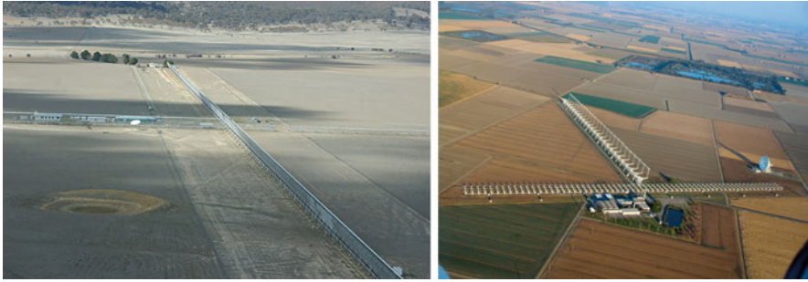
Fig. 2.3 Left: Aerial view of the Molonglo Cross Radio Telescope. The more visible arm in the picture is the 1.6 km east-west arm which intersects the north-south arm, also 1.6 km long, in the centre of the picture. (Courtesy of the University of Sydney Archives). Right: Aerial view of the Northern Cross Radio Telescope at Medicina comprising a single cylinder E-W arm 564 m long in the background, and a 640 m long array of 64 shorter cylinders as the N-S arm in the foreground. (Courtesy of INAF-Institute of Radio Astronomy)
