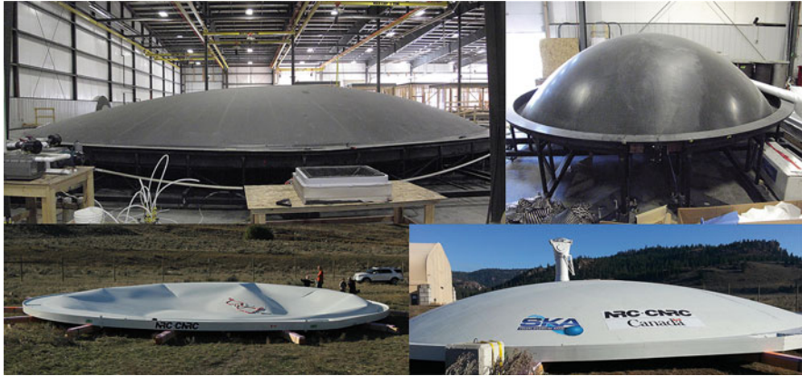
Fig. 6.16 Top Left: The mould for the DVA-1 main reflector ( 16 \times 18 m) under construction. Top Right: The DVA-1 mould for the sub-reflector (4 m diameter). Bottom left: The DVA-1 reflector unexpectedly becoming airborne and being abruptly halted by the rigging during helicopter transport. Credit: Gary Hovey. Bottom right: The reflector after being “popped back into place” and repaired. Credit: The National Research Council of Canada
