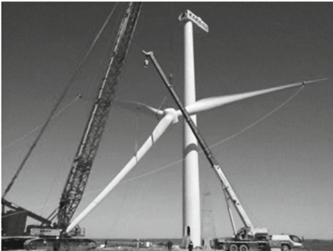
Fig. 1 Wind turbine hub lifting
