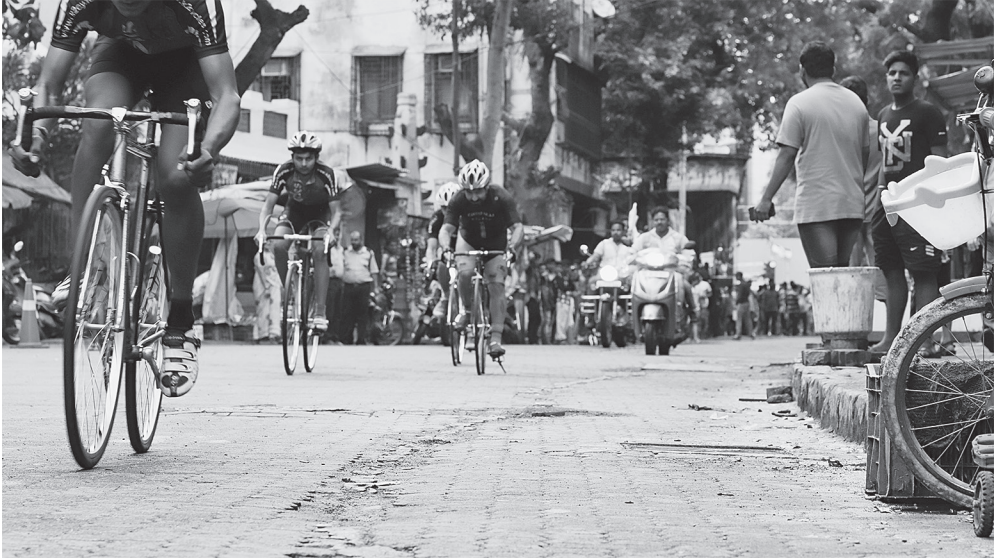
Participants in the annual Custom Point race, including Mirza Saaib Bég ( center ), navigating a street with uneven, cracked, and missing paver blocks.
