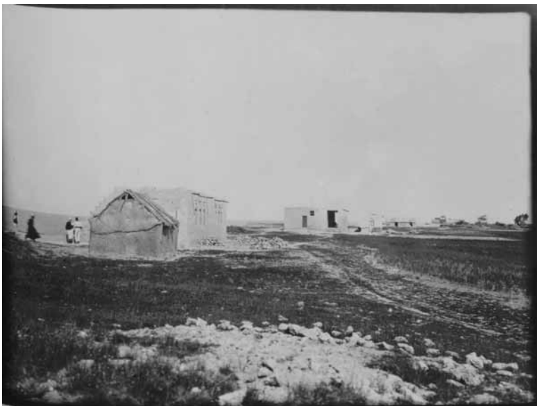
Figure 1.5 Bushehr quarantine station on the island of Abasak. The building in the foreground is the second-class block; the hut just beyond is the first-class block; and in the distance is the third-class hut of the disinfecting house. Confidential Report by Dr Theodore Thomson on the Sanitary Requirements of certain places in or near the Persian Gulf, &c. 12 July 1906. FO 368/37
