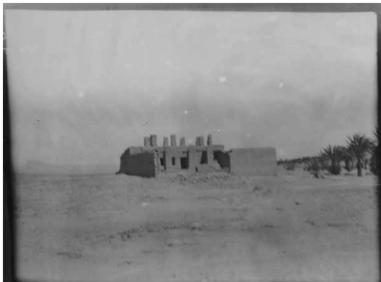
Figure 1.3 Jask quarantine station from behind. Confidential Report by Dr Theodore Thomson on the Sanitary Requirements of certain places in or near the Persian Gulf, &c. 12 July 1906. FO 368/37
