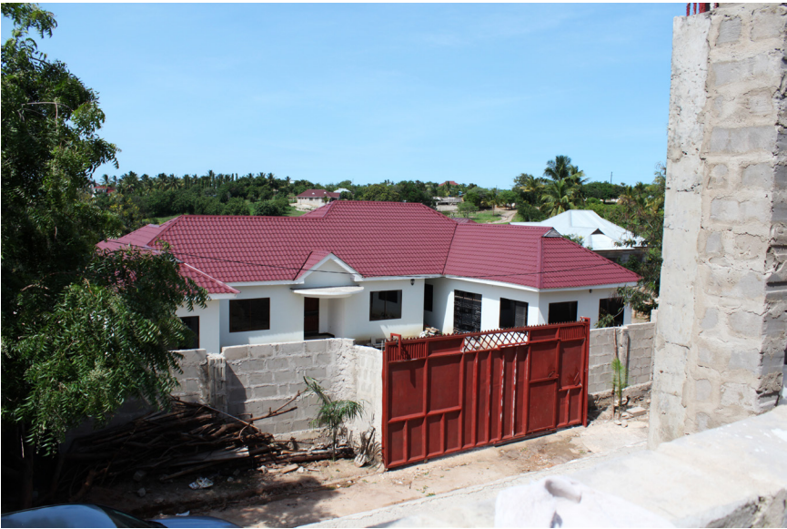
FIGURE 2. The same house in April 2015. Photo by author.
