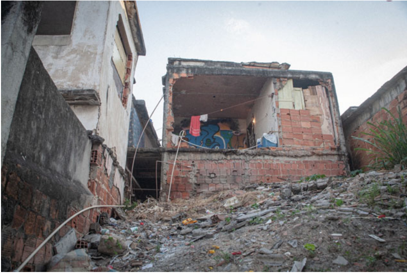
Fig. 8.1 A building in shambles in Alemão, April 2015
