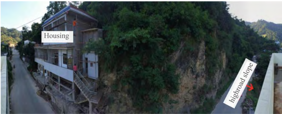
Fig. 4. The status of both sides of the highway
