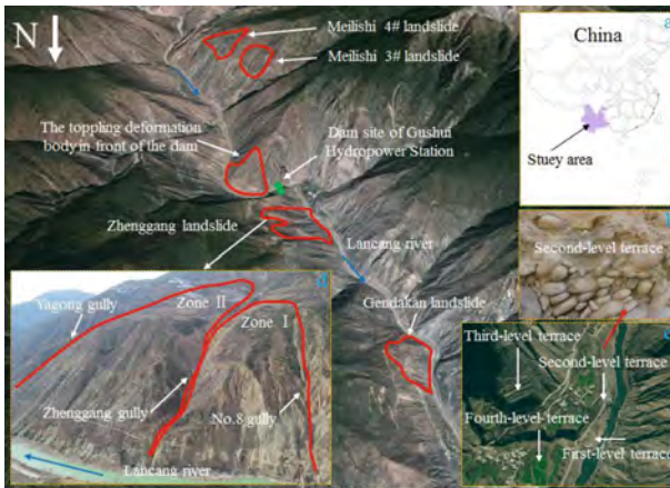
Fig. 2. The typical landslide in the study area (a. the location of Zhenggang landslide; b. Second-level terrace Pebble layer; c. First to fourth-level terrace; d. Full view of Zhenggang landslide).
