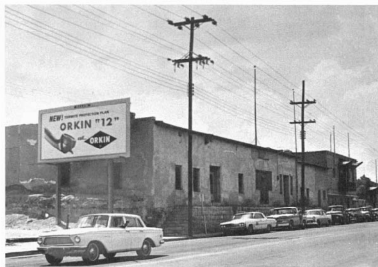
Figure 2.21. The Ying On compound as it appeared in 1968 prior to demolition: top , the Ying On Merchants and Labor Benevolent Association building erected in 1950 at 103 south Main Street; bottom , the western facade (Unit 2). The two nearest flagpoles were over the doorways of the meeting rooms of the Chee Kung Tong (Chinese Masons) and the Guomindang (Nationalist Party).
