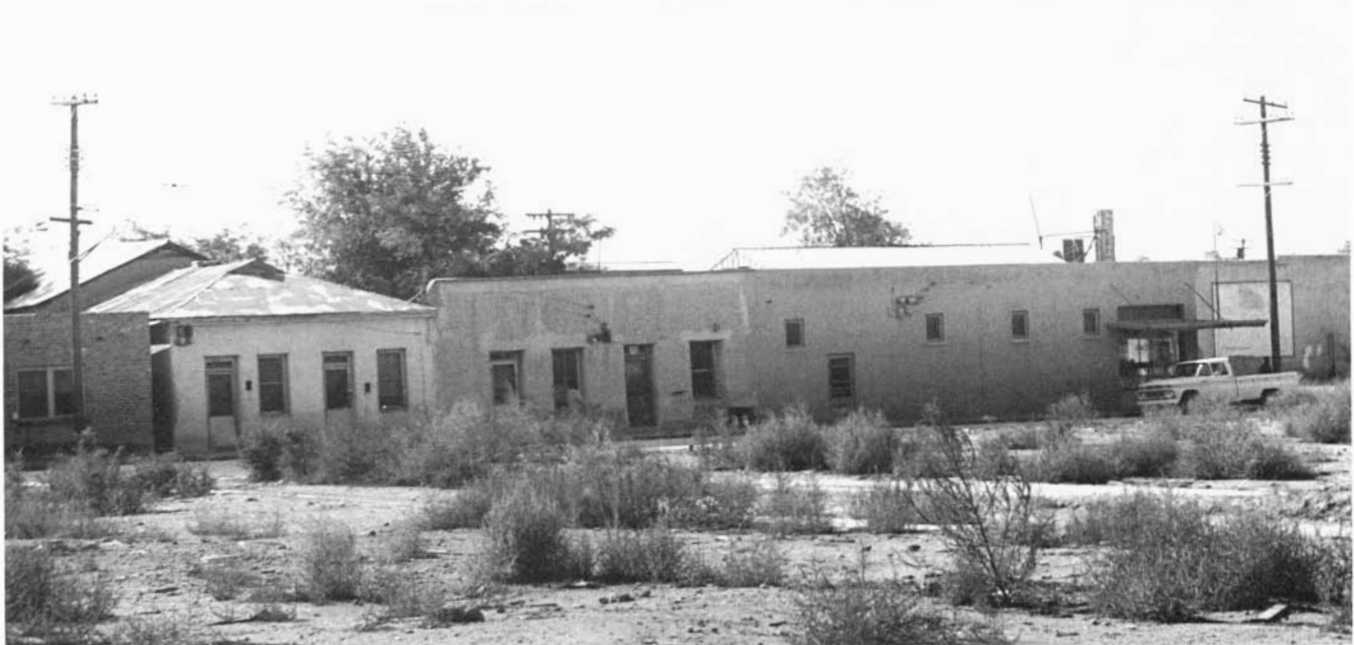
Figure 2.5. North facade of the Suey Yuen store and dwelling at the southeast corner of south Meyer Street and west McCormick Street. At the center of the view were two apartment rentals. The section of wall with four high windows and a large display window under a metal awning was the store that fronted onto south Meyer Street. (Arizona State Museum photo by D. Hsu.)
