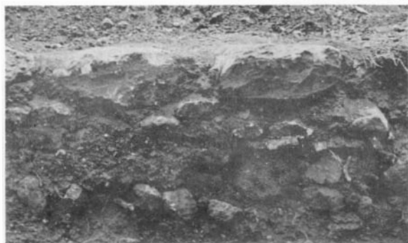
FIG. 43. Ruin B, Room 3, wall detail. Core-and-rubble masonry with mud-pebble-cobble veneer.
