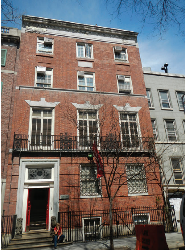
Fig. 2. China House, 2013. (Photograph by Jim Henderson, courtesy of Wikimedia Commons.)
