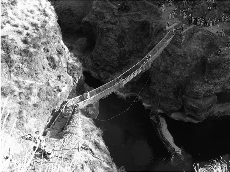
Figure 2.4 The old bridge flows down the stream of the Apurimac River – with the weaving of a new one, another cycle begins Source: Photo by the Author.
