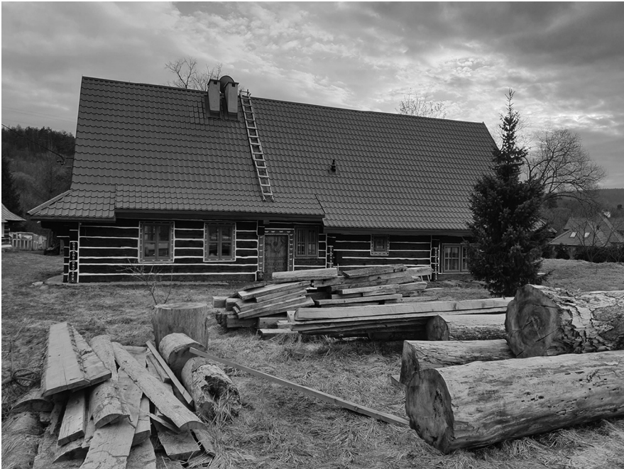
Figure 14.2 A chyża house undergoing restoration
