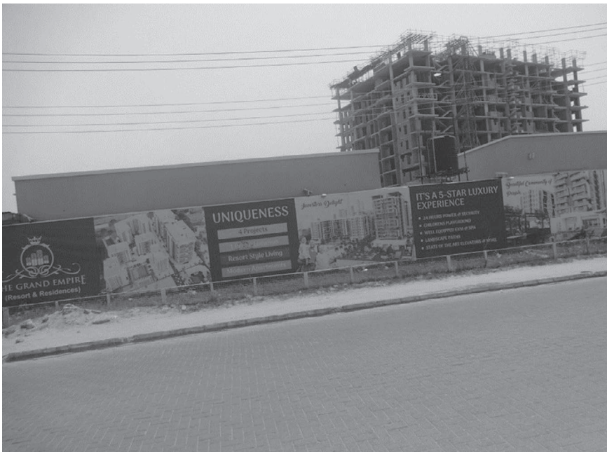
Figure 9.1 Luxury apartments under construction in Lekki, Lagos.
