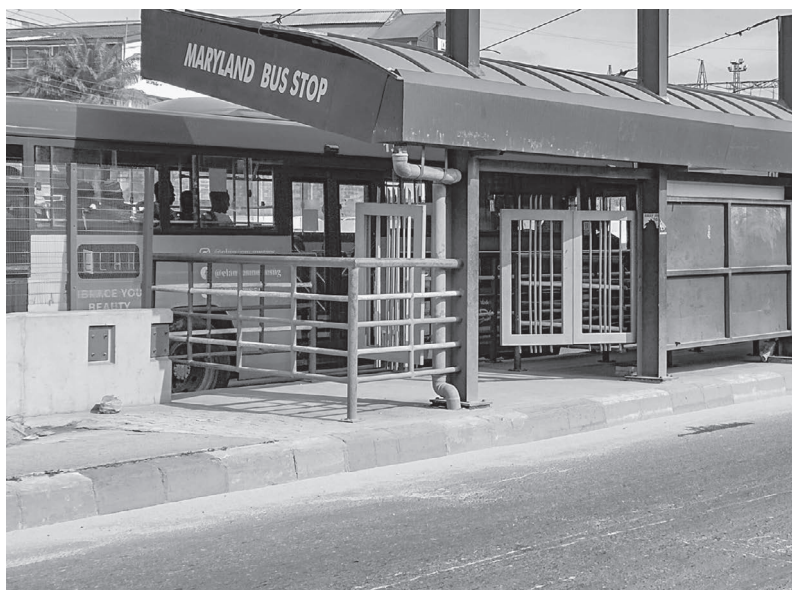
Figure 5.2 A BRT bus stop lacking disability access.
