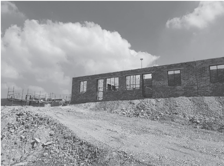
Figure 8.4 Apartment block construction as of early 2022.
