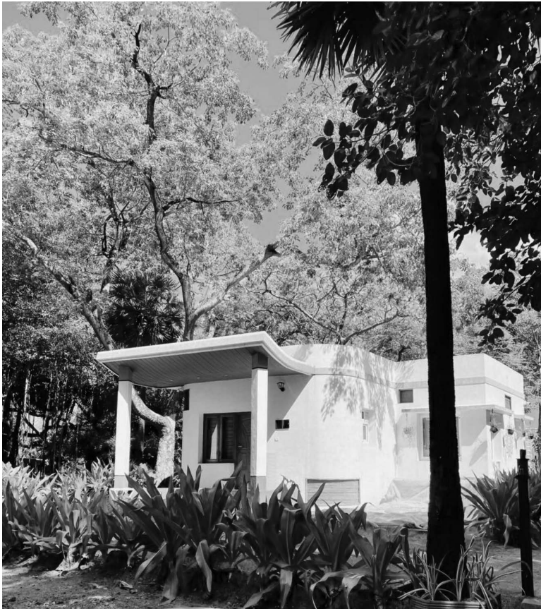
FIGURE 3.7 3D-printed concrete house at IIT Madras.
