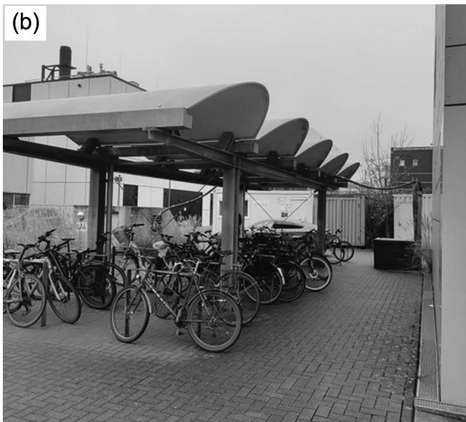
FIGURE 3.4 Application of TRC: (a) TRC facade construction in Mumbai, India, by Raina Industries [57]; (b) cycle shed made of TRC shell elements at Institute of Textile Technology at RWTH Aachen University, Germany [58].
