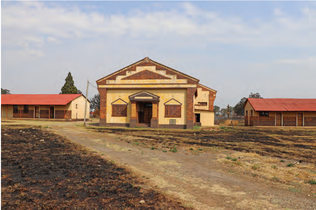
Figure 9.2 Bonner Hall, Wilberforce Institute, Evaton, 2021. Photograph: Nomusa Makhubu.
