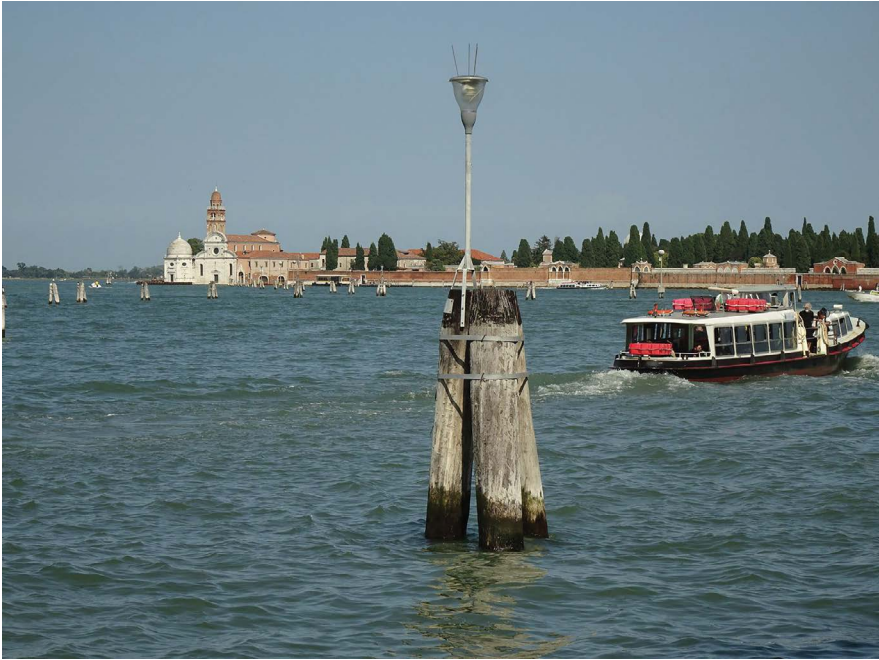
Figure 3.2 Grid tripods ( briccolle ) as part of the Venice Lagoon navigable landscape
