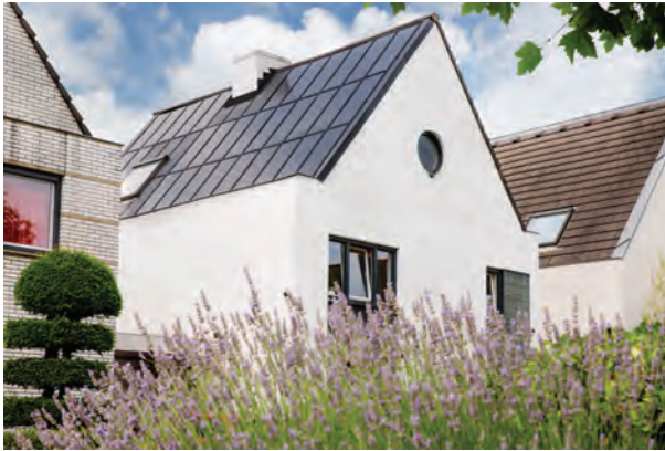
FIGURE 5.13 House renovated with a full roof BIPV solution of Beausolar. Around the chimney and skylight dummy pieces are installed to retain a homogeneous appearance. (From Beausolar, Beausolar Project Webpage. https://beausolar.eu/projecten/ , 2019.)
