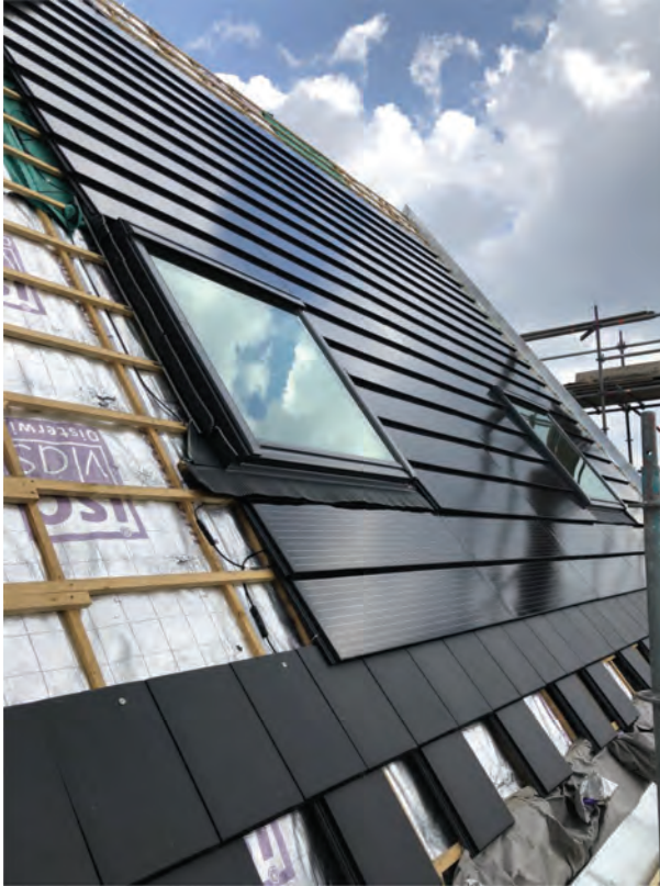
FIGURE 5.16 Solinso Mystiek solar roof tile combined with skylights and standard flat roof tiles. (From Solinso, Solinso brochure 2018: Mystiek Zonnedakpannen, https://www.solinso.nl/images/downloads/Brochure-Solinso-2018-.pdf , 2018b.)
