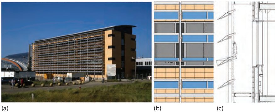
FIGURE 5.18 (a) BIPV shading system installed on ECN office building 31, (b) front side sketch, (c) schematic drawing of the mounting system of the shading lamellas. (BEAR architects, http://bear-id.com/projects/ecn-building-42/ , 2019.)
