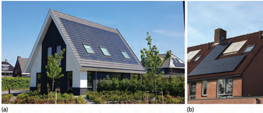
FIGURE 5.1 (a) BIPV: PV roof tiles integrated into the roof and hardly visible. When PV modules are removed, new tiles must be placed to maintain water tightness of roof. (Solinsko 2018b); and (b) BAPV: PV modules are placed on top of the roof tiles. PV modules can be removed without losing other roof functions than electricity generation. (©W. van Sark)
