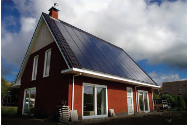
FIGURE 5.14 A house in the north of the Netherlands, equipped with Viridian Solar's Clearline Fusion. An in-roof PV system with standard-sized solar modules.
