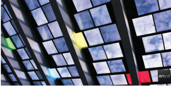
FIGURE 5.12 Skylight on the historic food market of Bejar, Salamanca (Spain). Amorphous silicon modules with varying degrees of transparency are combined. (From Onyx https://www.onyx-solar.com/bejar-market , 2019b.)
