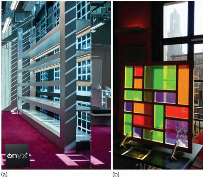
FIGURE 5.10 (a) Curtain wall equipped with relatively small crystalline silicon cells with large spacing between the cells (Balenciaga store, Miami, FL, USA) (From Onyx Solar, https://www.onyx-solar.com/balenciaga-store-miami , 2019a.); and (b) photograph of the 1 m 2 Electric Mondrian™ with the Utrecht Dom tower in the back. (From van Sark, W. et al., Solar RRL , 1, 1600015, 2017.)
