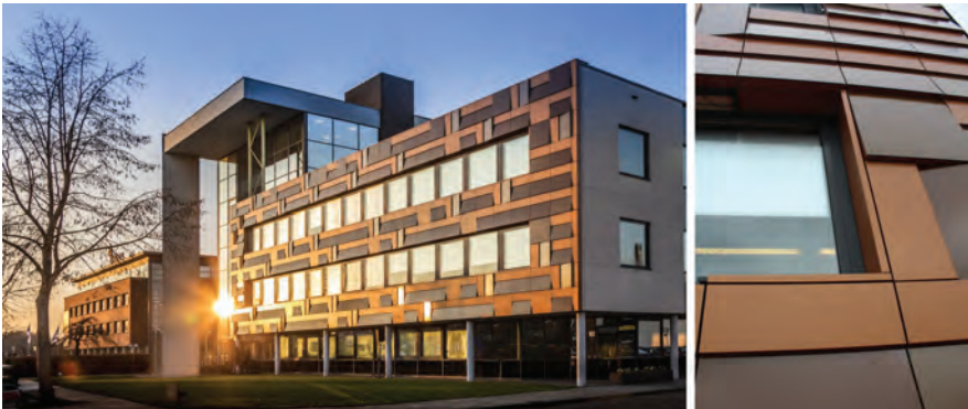
FIGURE 5.7 Kuijpers building Helmond (The Netherlands), the south façade is equipped with 177 custom-made BIPV elements. A consortium consisting of Kuijpers, Studio Solarix, Sorba, and Kameleon Solar was responsible for the design and realization of this building.
