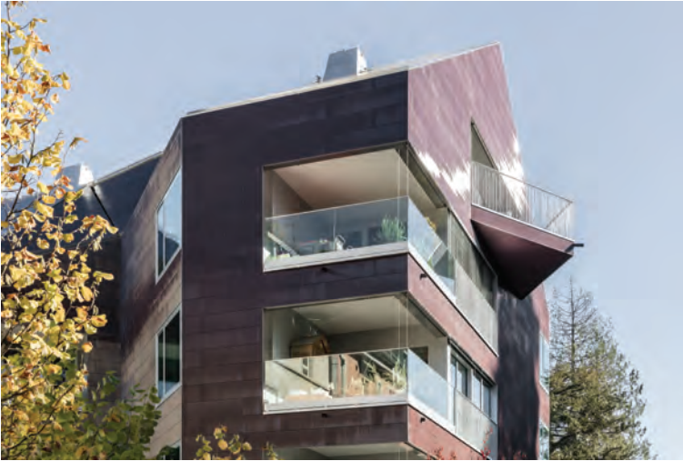
FIGURE DC-5.5 A detail of the glittering effect, similar to the water surface of the lake, given by the use of the PV modules. (Courtesy of Beat Bühler, photographer Zurich, Courtesy of Huggenbergerfries Architekten.)
