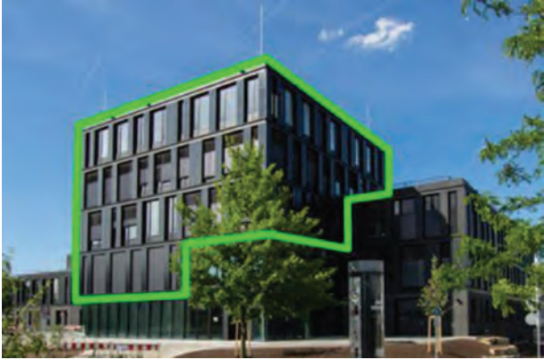
FIGURE 5.21 PV Façade at the ZSW laboratory and office building in Stuttgart (Germany). The green line indicates the building block on which BIPV elements are installed. (From Geyer, D et al., Research project CIGS-Façade, PV façades—chances and limits, Proceedings of the 35th European Photovoltaic Solar Energy Conference , pp. 1805–1808, 2018.)
