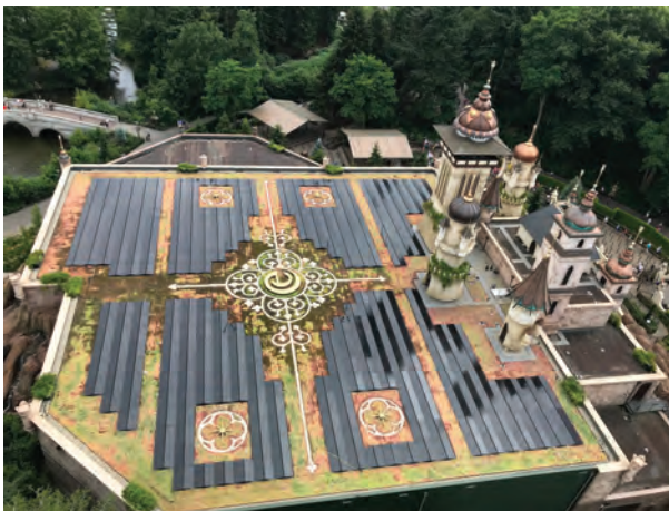
FIGURE 1.3 A well-integrated PV system looking like a French garden in the Efteling in the Netherlands. (Courtesy of Angèle Reinders.)
