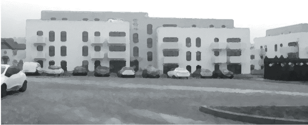
Figure 2. Eco-town at the finishing stage.
