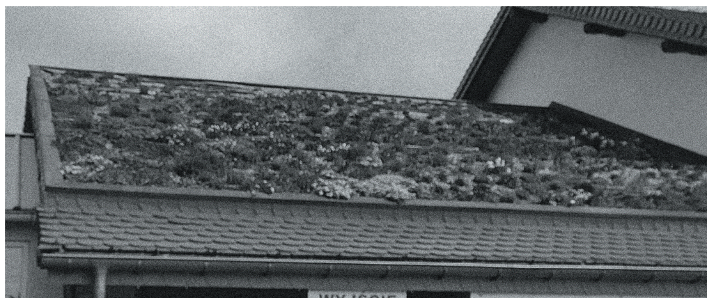
Figure 1. The usage of green space within a commercial facility in the Silesian province.
