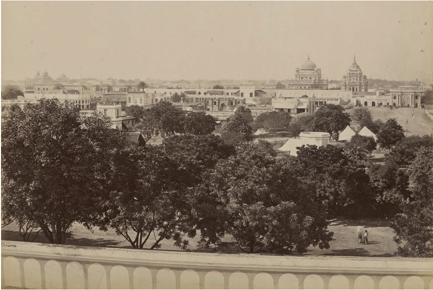
Figure 8.8 China Bagh seen in a photograph by Samuel Bourne. 1865–66.
