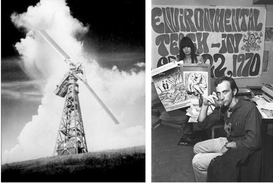
Fig. 8.1 (Left) The Smith-Putnam wind turbine built on Grandpa’s Knob in Castleton, VT, which commenced operation in October 1941. (Source: Putnam, 1948) (Right) Denis Hayes, organizer of the first Earth Day in 1970. (Source: AP)
