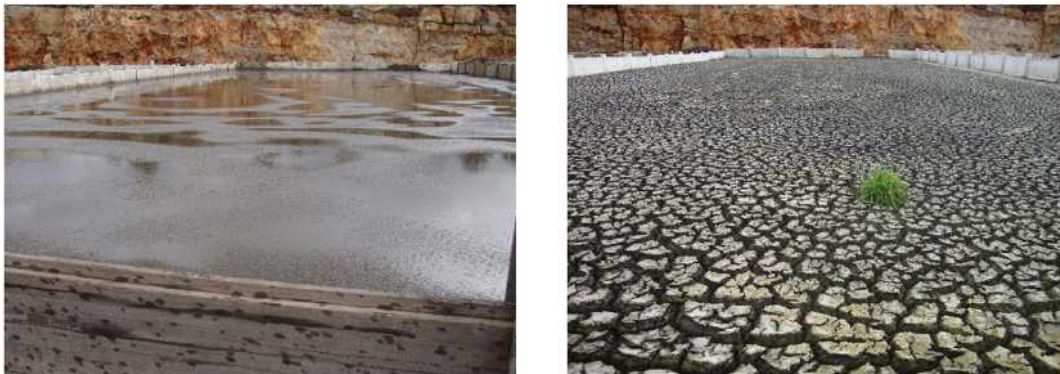
Figure 6.13 Sludge-drying bed in a municipal STP containing fresh sludge (left) and with dehydrated sludge (right).
