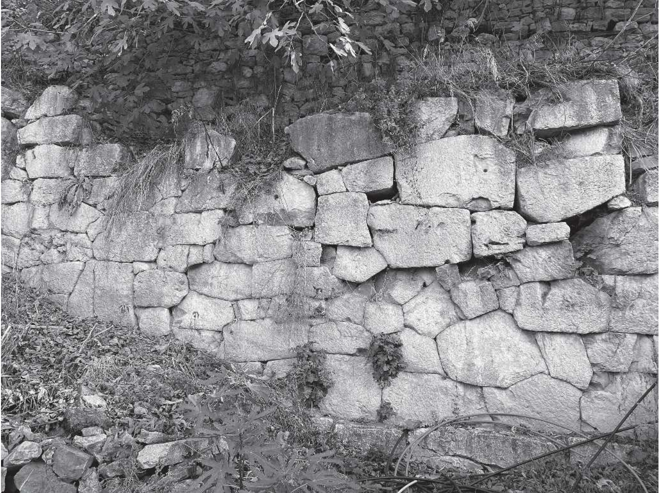
Figure 16 Fortification wall in polygonal masonry behind the dimarcheio of Domokos. © Greek Ministry of Culture and Sports – Organization for the Management and Development of Cultural Resources.
