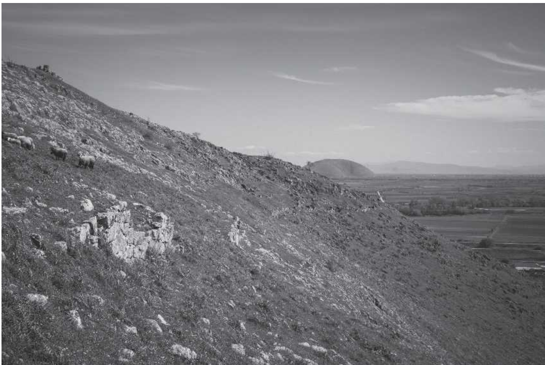
Figure 47 The fortifications in the southwest slopes of the Vigla hill, looking southeast. At horizon, Stroggylovouni at Vlochos. © Greek Ministry of Culture and Sports – Organization for the Management and Development of Cultural Resources.
