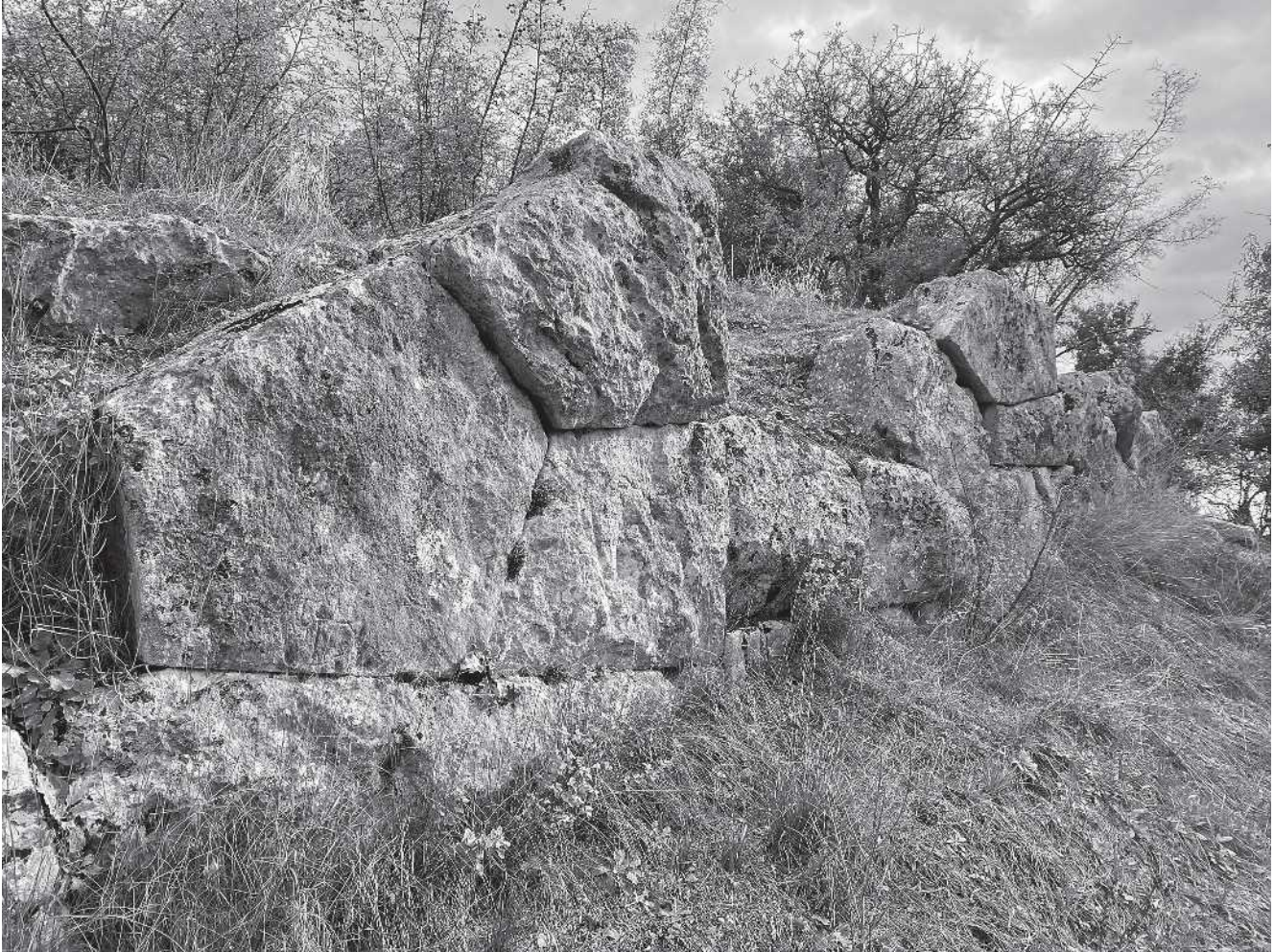
Figure 78 Fortification wall in polygonal masonry, western slope of the Skoumpos hill. © Greek Ministry of Culture and Sports – Organization for the Management and Development of Cultural Resources.
