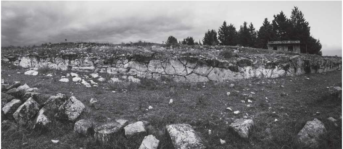
Figure 73 Panoramic view of fortification wall in polygonal masonry at the akropolis of Kierion. © Greek Ministry of Culture and Sports – Organization for the Management and Development of Cultural Resources.
