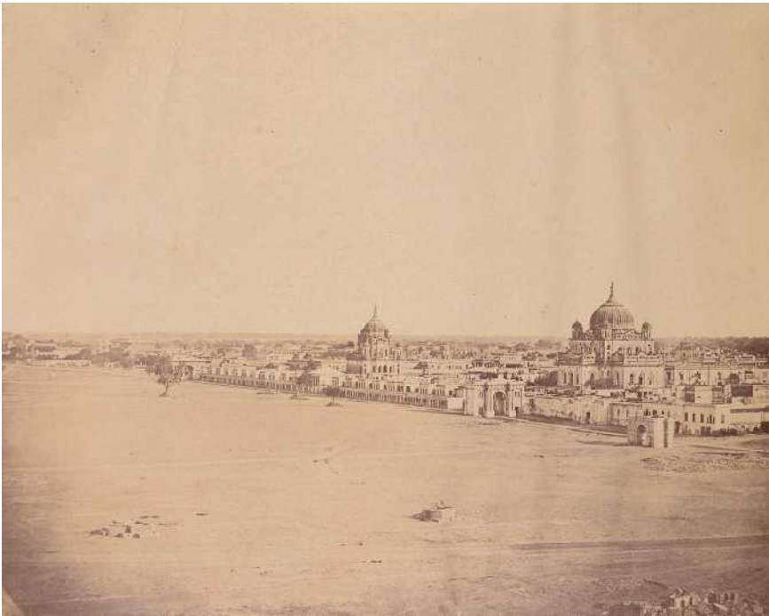
Figure 8.7 China Bazaar seen in a photograph by John Christian Andrew Dannenberg. c1867.
