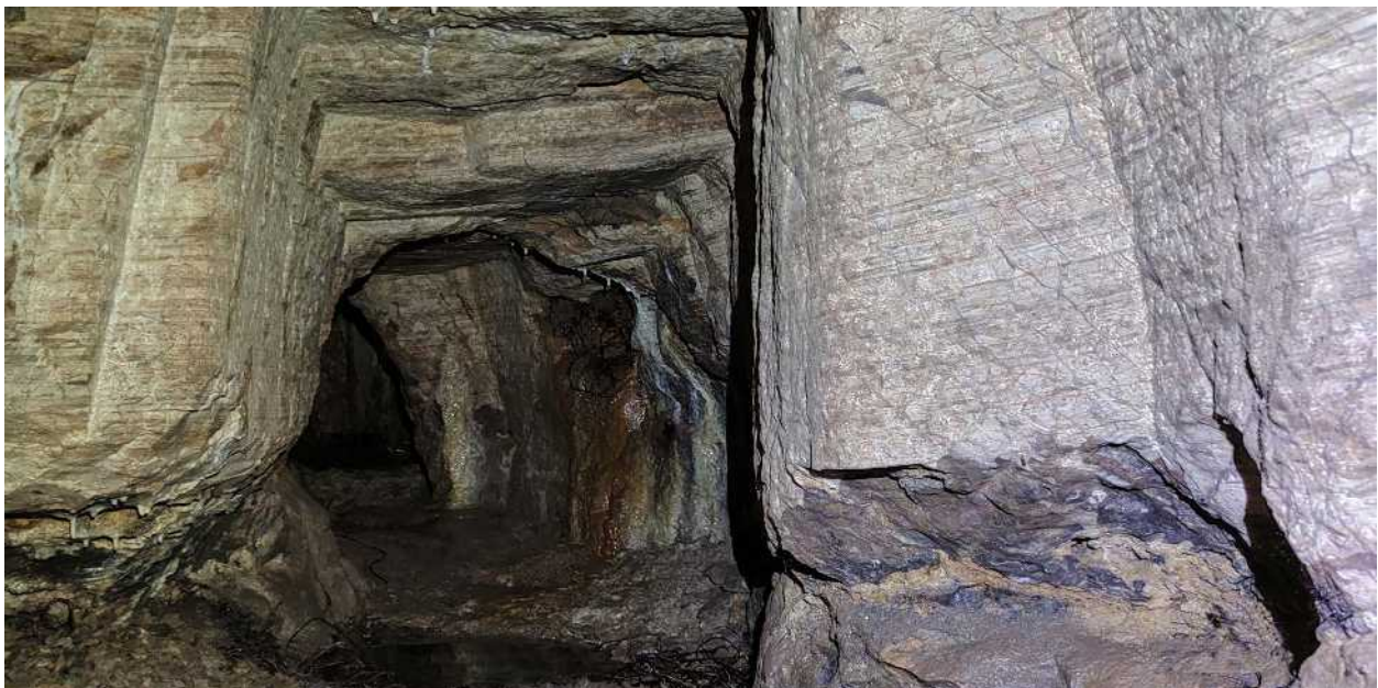
Figure 1. A mining underground work in the proximity of Esperanza area in Lavreotiki. Tiny residues of a galena vein are observed at right. Cerussite and galena ore was extracted exhaustively at this place, leaving behind a vast room inside marble. A drift continues ahead, following the vein, in search of other ore concentrations.
