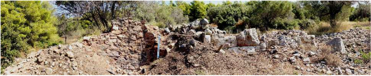
Figure 3. The remains of the roasting furnace at left, which formed a complex along with two or three other furnaces, now completely ruined (at right).
