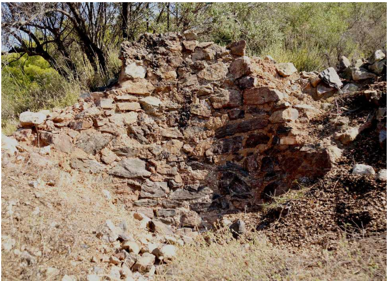
Figure 2. The remains of the Roasting Furnace discovered at Dimoliaki-Lavreotiki. The furnace was used in the Hellenistic-Early Roman period for roasting of galena.
