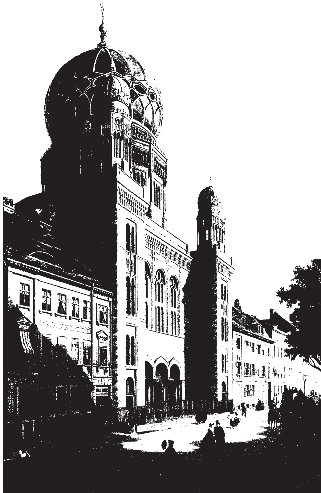
Fig. 5 Facade of the Oranienburger Straße synagogue, inaugurated in Berlin in 1866. Photograph from Märkisches Museum, Berlin.
